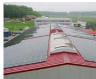
Industrial construction D Built in 2009 Power 105 kWp
