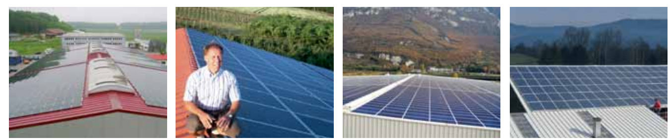
Industrial construction D Built in 2009 Power 105 kWp
