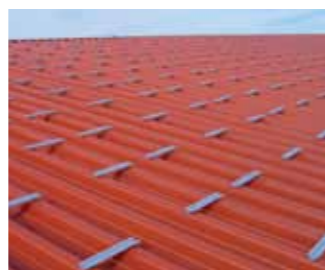
Equestrian hall D Built in 2008 Power 55 kWp
