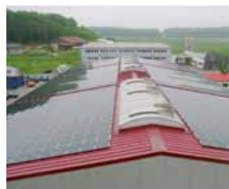
Industrial construction D Built in 2009 Power 105 kWp
