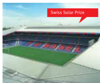
St. Jakob Stadium Basel Built in 2001/2004 Power 150/200 kWp
