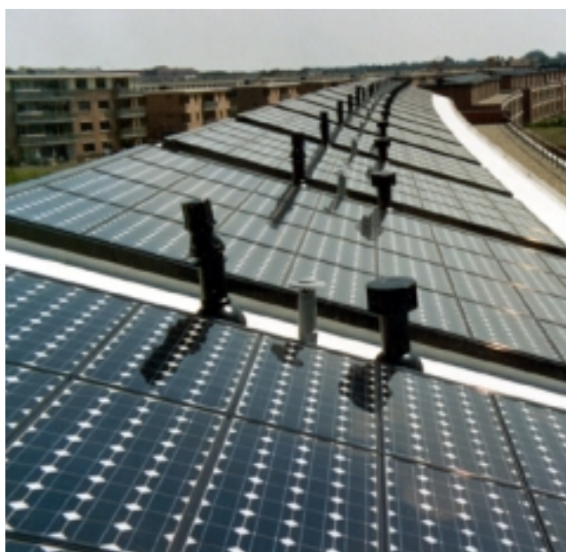
Photo 3: Roofs of Housing Scheme at Amersfoort, Holland
