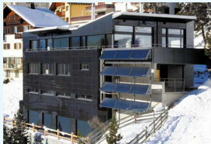
Front mounted rear-ventilated glass facade with frameless 3S Swiss Solar Systems solar laminates in St. Moritz (CH).
