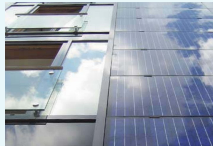
Custom 3S Swiss Solar Systems solar laminates for full facade integration in Landsberg (D).
