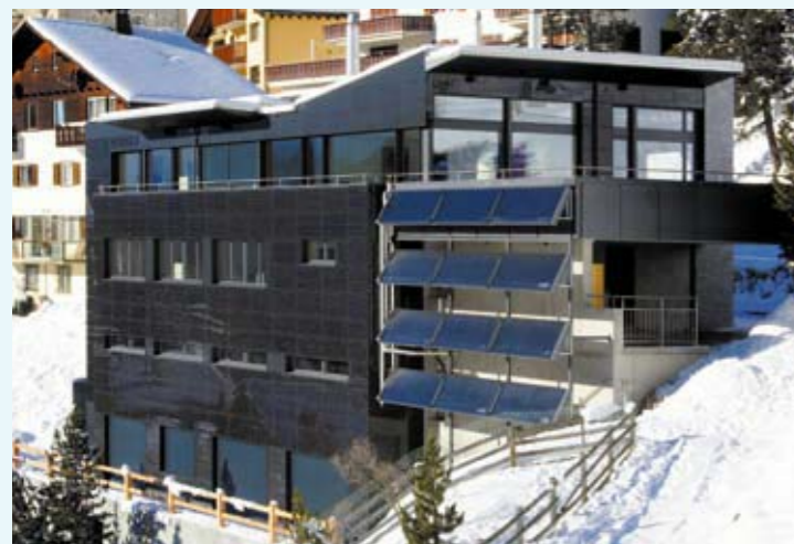
Front mounted rear-ventilated glass facade with frameless 3S Swiss Solar Systems solar laminates in St. Moritz (CH).
